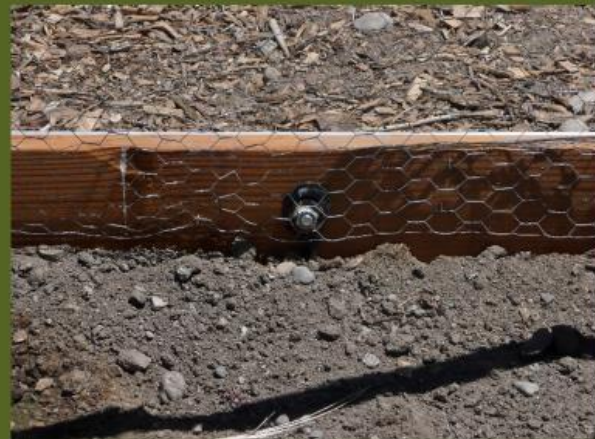
Added corkscrew anchors embedded in concrete
