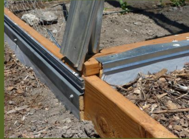
Added flashing over R max
