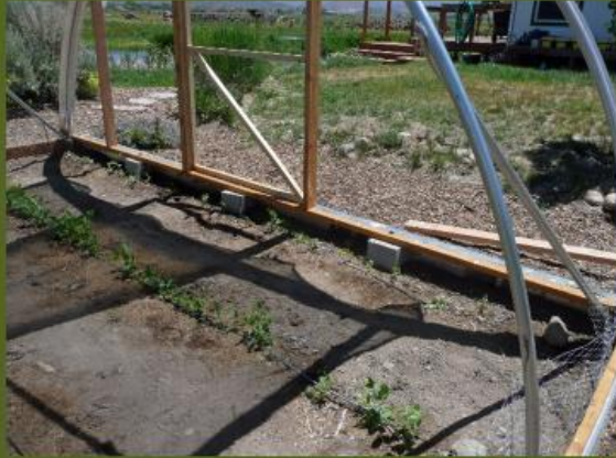
Added cinder block anchors on end walls
