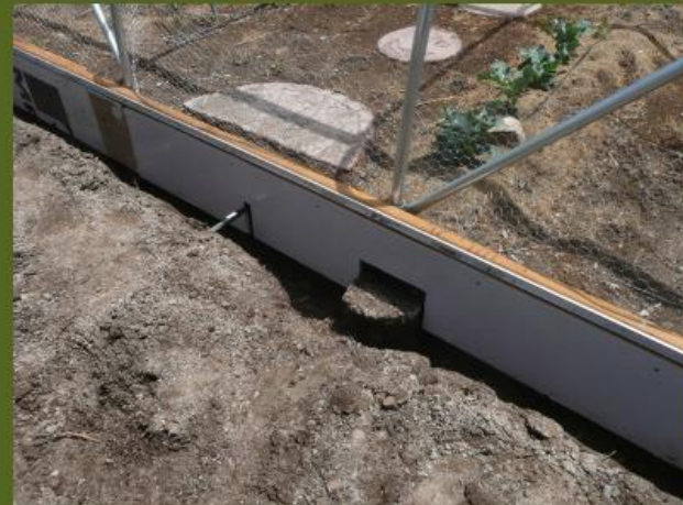
Added R max insulation Below ground level
